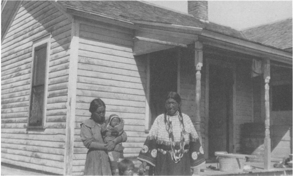
Figure 1. Photograph from the Industrial Survey, Rosebud Reservation, 1923. Washington, DC: National Archives and Records and Administration.
